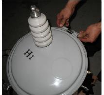
A recommended procedure for opening the transformer is to first bring the interior of the transformer to atmospheric pressure by venting the automatic pressure relief valve furnished on all CCHN transformers. The cover band may then be removed. Natural rubber hose should not be used in the transfer of oil. The correct oil level at 25°C is marked on the inside of the tank.
